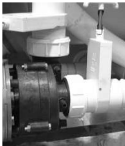
Slice Valve and Pump Union
