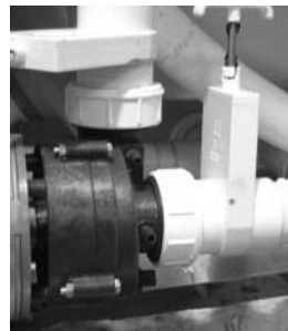
Slice Valve and Pump Union
