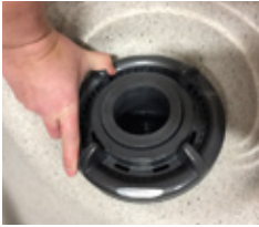
Twist Lock Ring Counter-clockwise to Remove Floater
