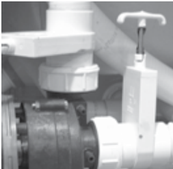
Slice Valve and Pump Union
