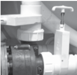
Slice Valve and Pump Union
