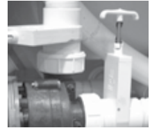
Slice Valve and Pump Union
