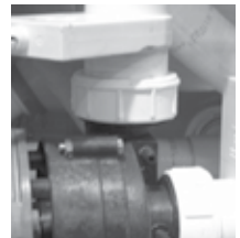
Slice Valve and Pump Union
