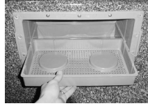
Pull Up on Plastic Skimmer Plate to Remove
