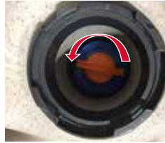
Turn Filters Counter-clockwise to Remove
