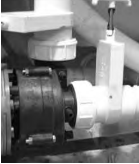
Slice Valve and Pump Union
