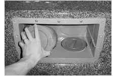
Turn Filter Counter-clockwise to Remove
