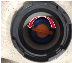
Turn Filters Counterclockwise to Remove
