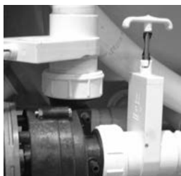
Slice Valve and Pump Union
