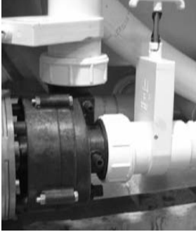
Slice Valve and Pump Union
