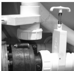
Slice Valve and Pump Union
