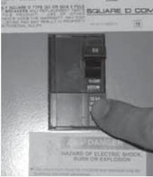
*\*The GFCI should be located in a weather proof box close to the spa, but no closer than 5 ft.*
