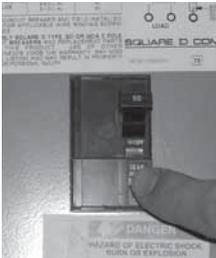
The Ground Fault Circuit Interrupter (GFCI) is required, by NEC code (National Electrician Code), for your protection. The tripping of the GFCI may be caused by a component on the spa or by an electrical problem. Such electrical problems include, but are not limited to, a faulty GFCI breaker, power fluctuations, or a miswire. It may be necessary to contact an electrician if your local dealer recommends doing so.
