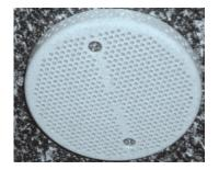
With the power to the spa off, remove the two screws holding the screen in place. Soak the screen in white vinegar and rinse thoroughly with water.
